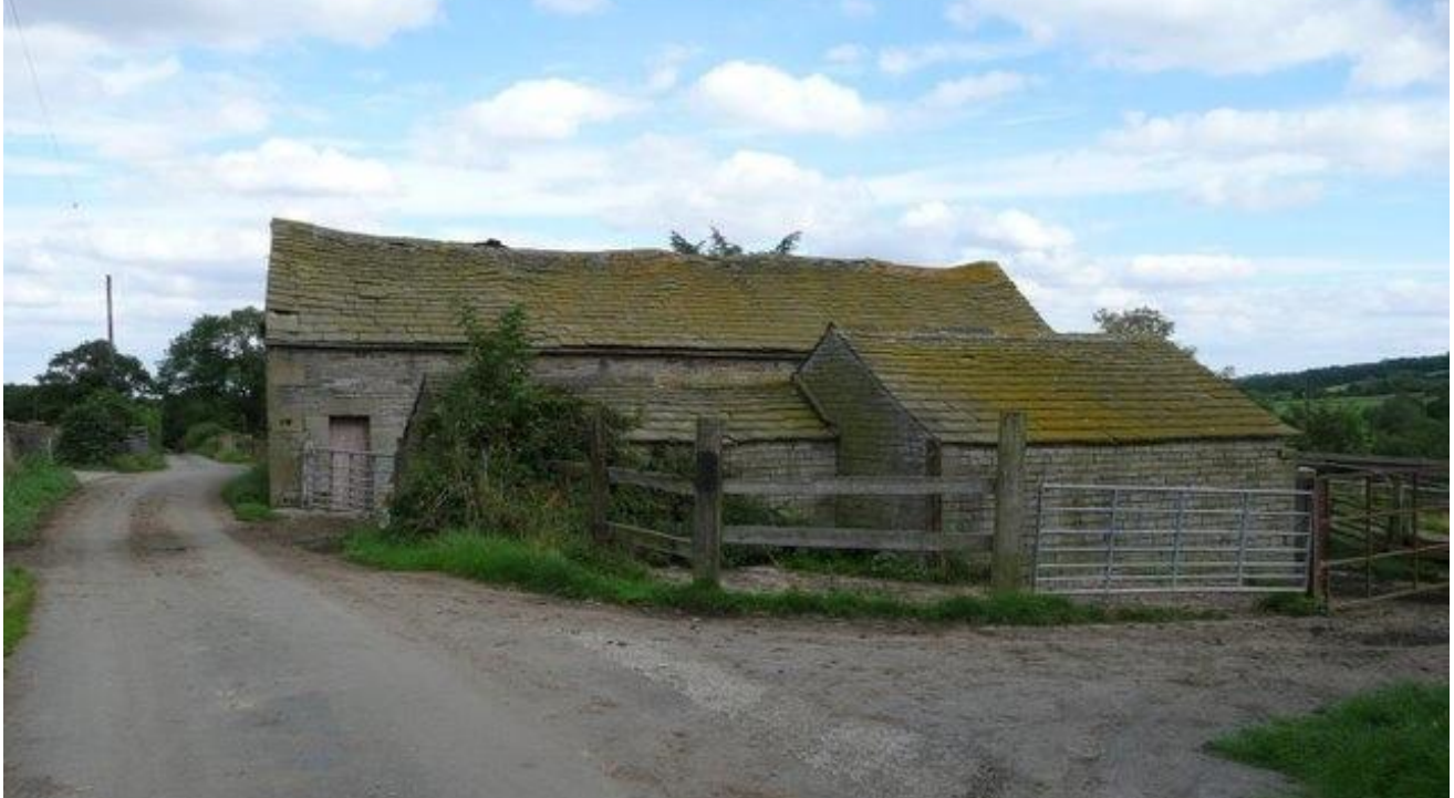
Sagging roof - the top of the roof is not a straight line, the middle dips down which indicates roof damage.
