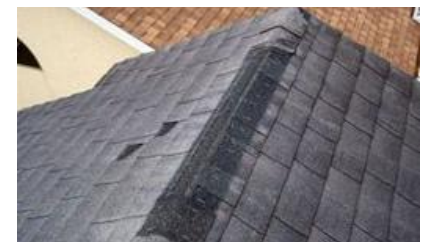
Hip and ridge cap lifting
