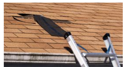
Missing shingles
