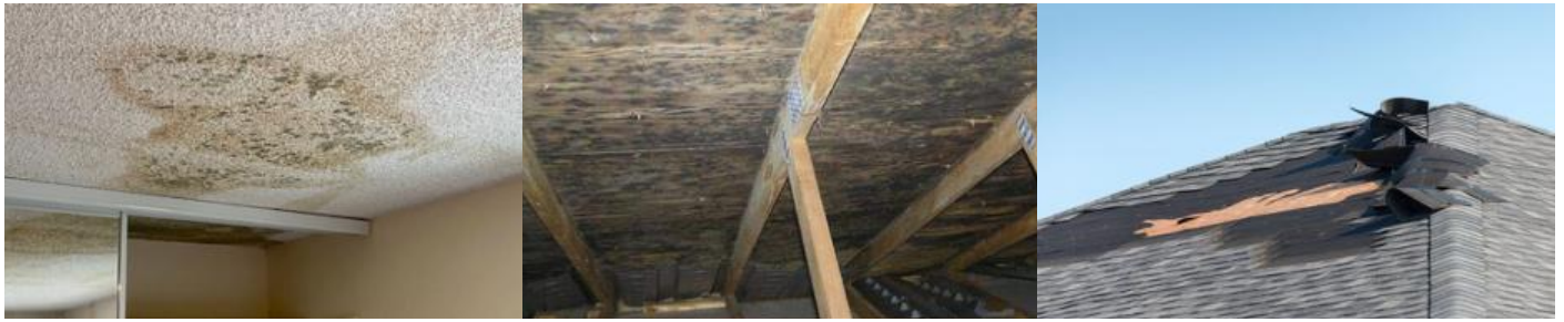
Water stains, black marks, and missing shingles are all indicators of roof leaks.
