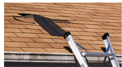
Missing shingles
